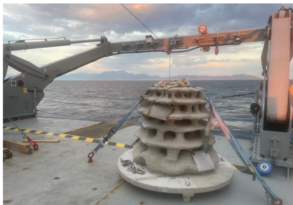
Photo of an artificial "ecoreef" structure positioned at the stern of the ship and ready to be placed on the seabed (Credits: Paolo Montagna)
