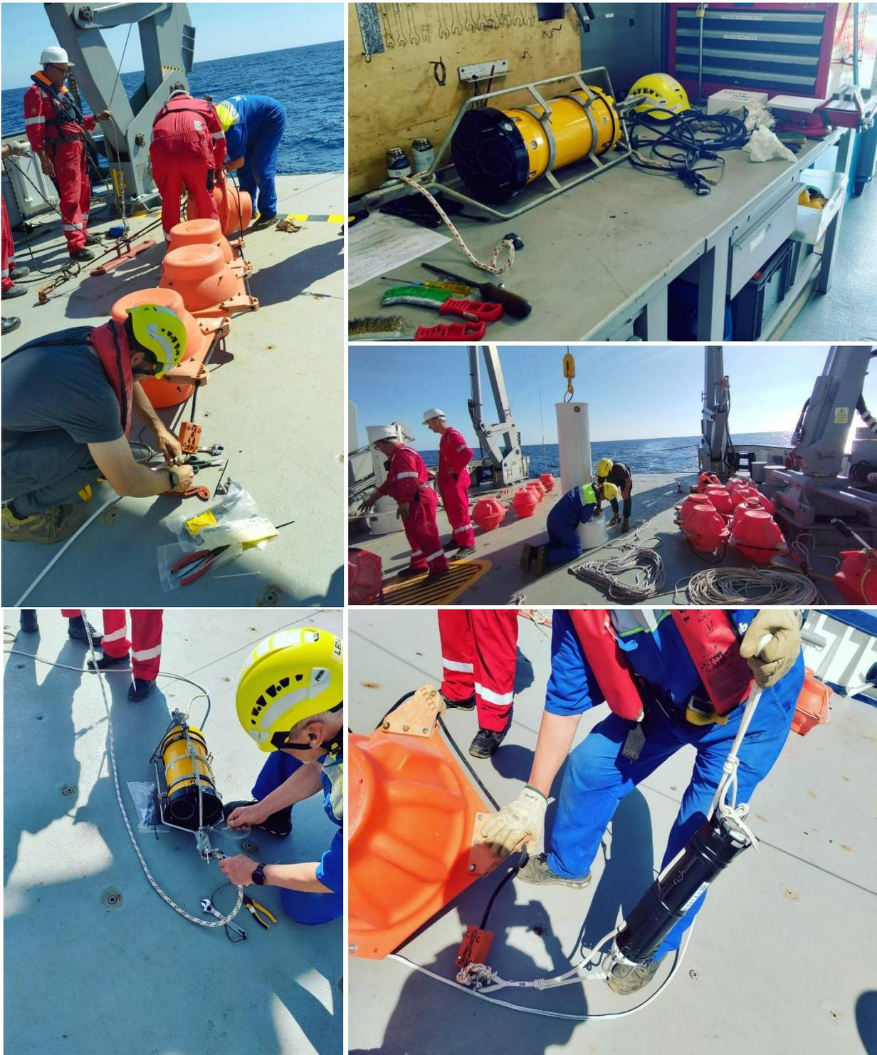
Figure 9.- Mooring preparation and deployment
